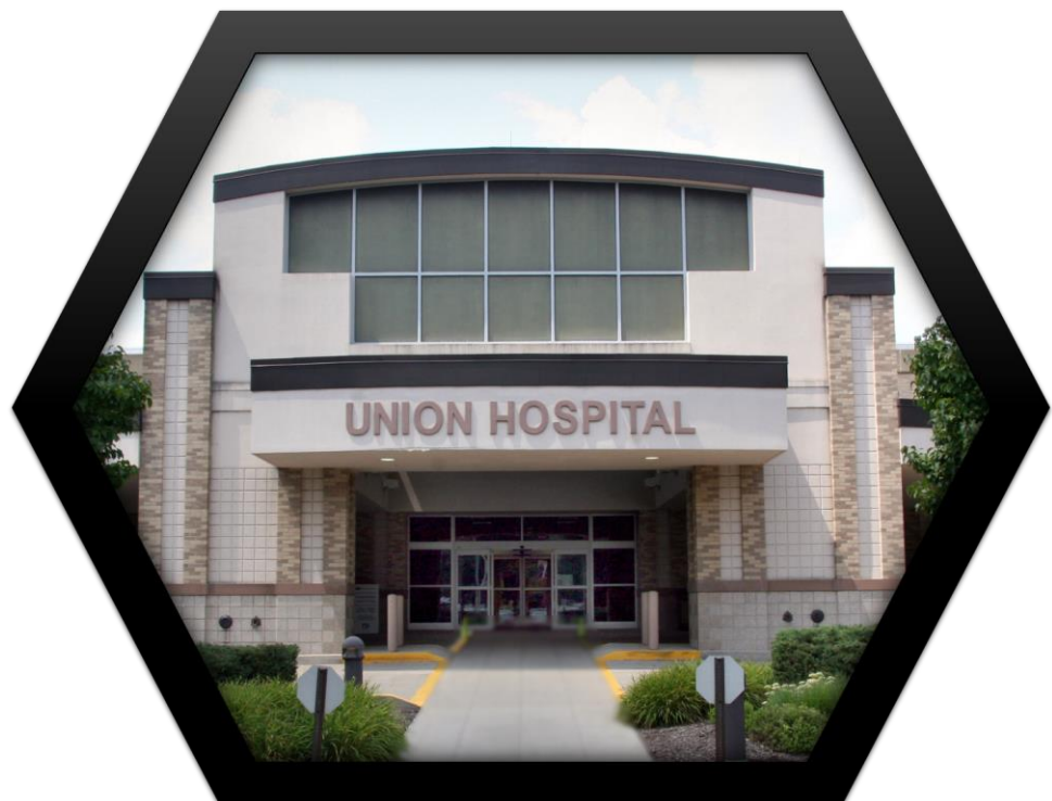
Union Hospital Dover, Ohio
